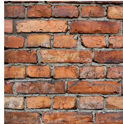
RECLAIMED BRICK - REAR WALL
