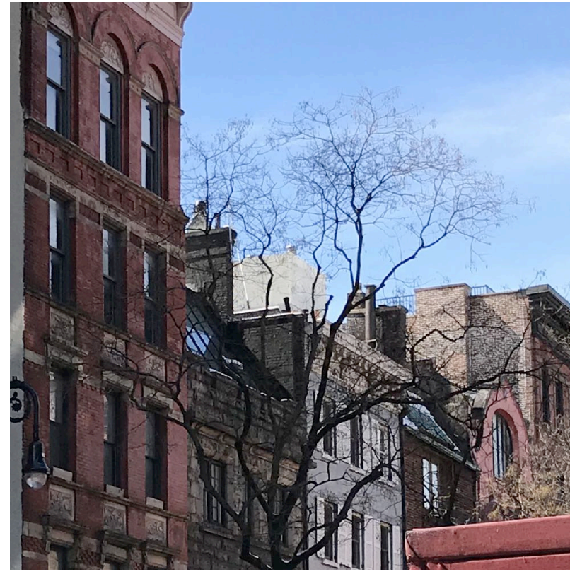
3. EXISTING VIEW 1 - DETAIL
